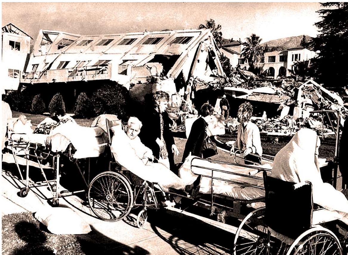
The VA hospital collapses in the Sylmar earthquake – picture ran in the Los Angeles Times on Feb. 10, 1971.
